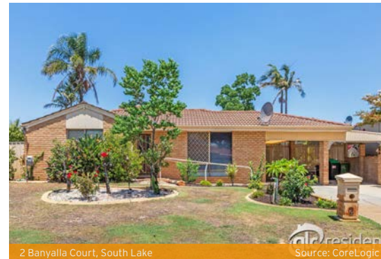
2 Banyalla Court, South Lake
