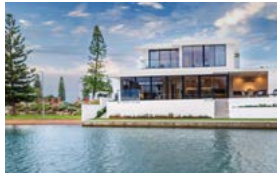
66 Martin Court, West Lakes Source: realestate.com.au
