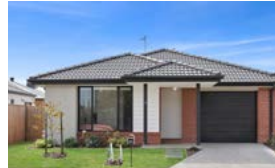
31 Robinson Street, Armstrong Creek
