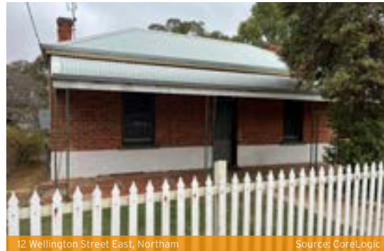
12 Wellington Street East, Northam
