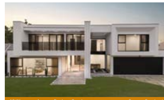
62 Wiregrass Avenue, Denham Court
