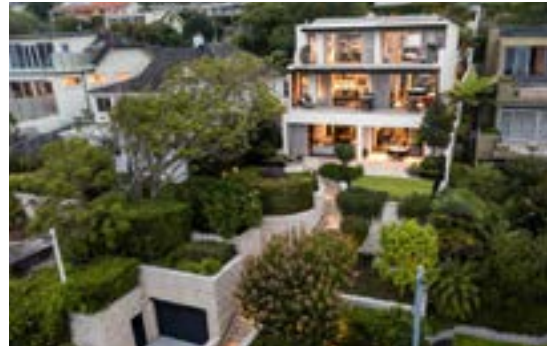
46 The Grove, Mosman Source: realestate.com.au
