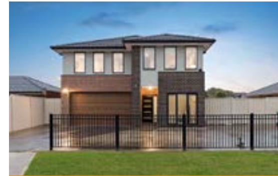
42 Delbridge Drive, Sydenham
