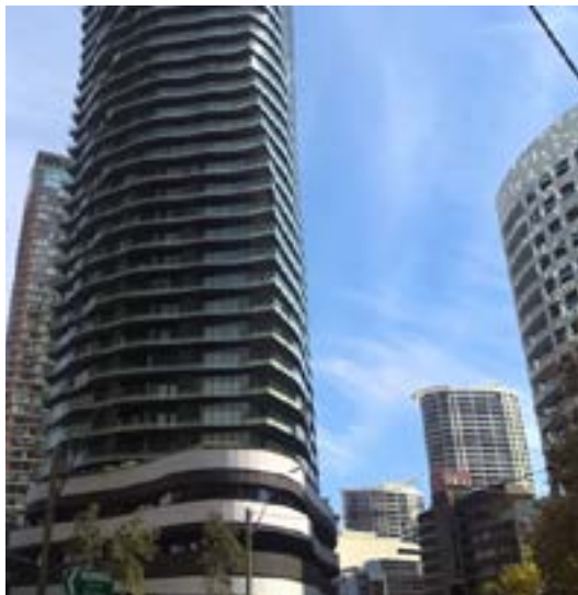
This development in St Leonards is typical of mixed use buildings with ground floor retail Source: Herron Todd White
