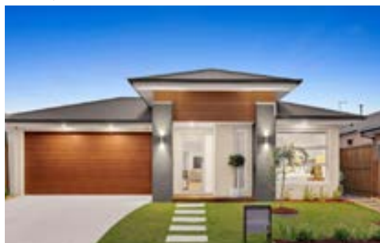
Cropping Street, Clyde North
