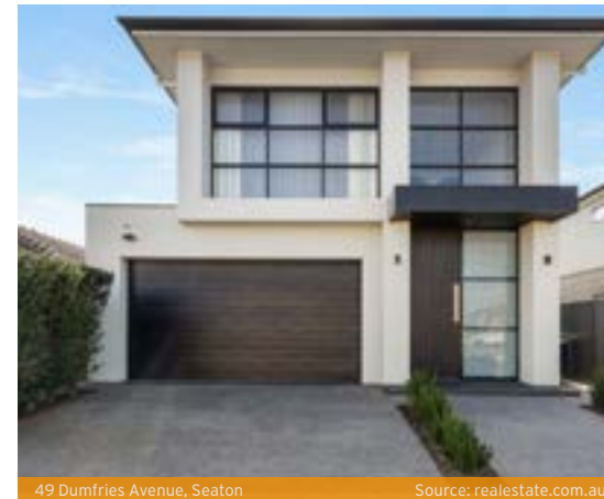
49 Dumfries Avenue, Seaton Source: realestate.com.au
